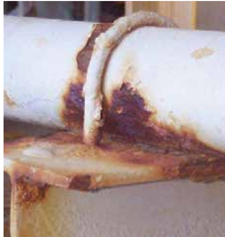
Above, the result of crevice corrosion on a pipe. Trapped moisture has caused substantial wall loss that could result in catastrophic failure.
